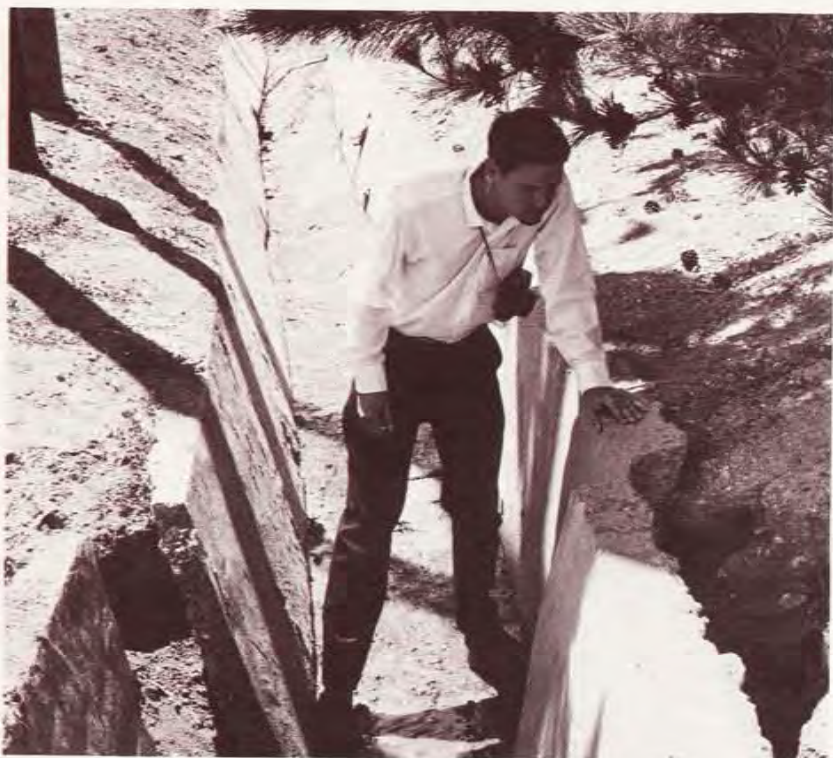
Dr. Robert D. Nason, in charge of NOAA's field studies of fault creep, checks the offset of a concrete-lined irrigation ditch at the Cienega Winery, where this non-seismic fault movement was first identified.
