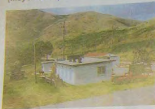
Nike site Visitor Center/Sentry building, portable radar systems. (Halsey)
