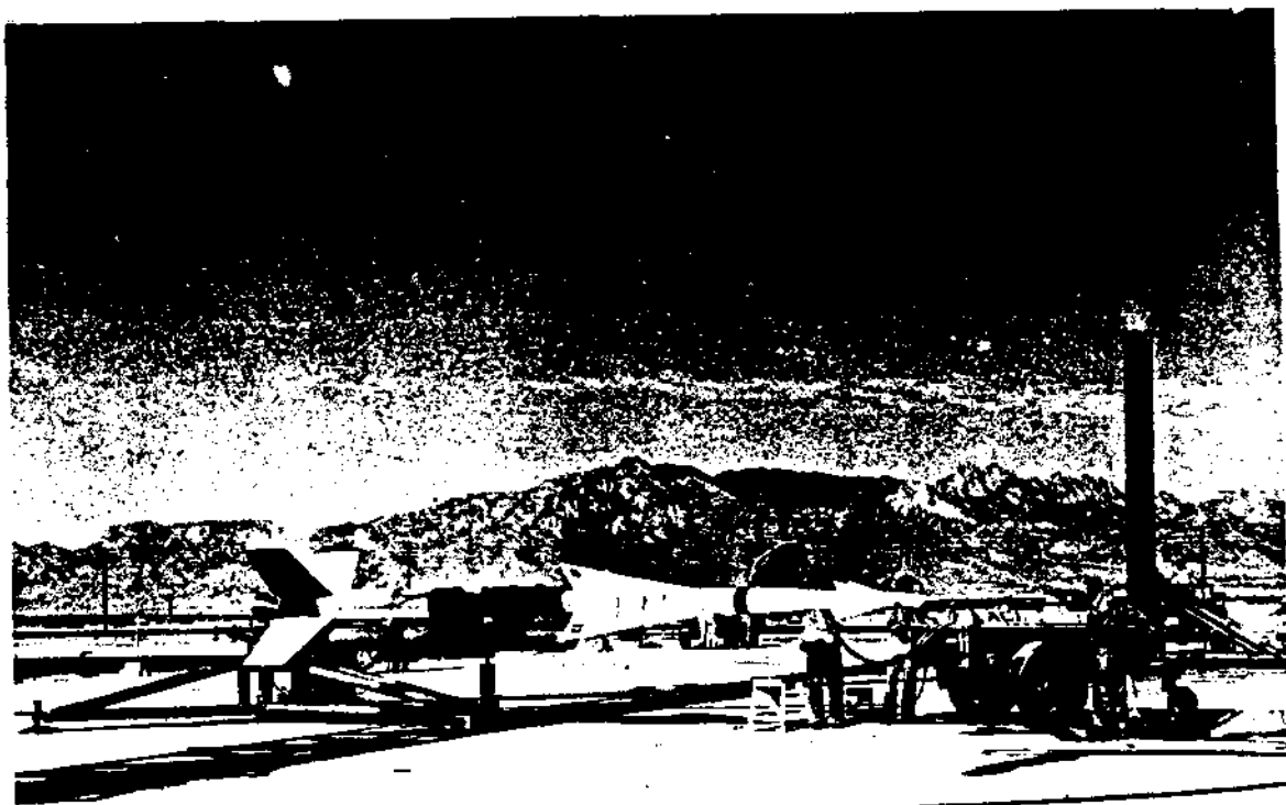
Figure 10. Oxidizer Fill, Round 14, Missile 47-17 (29 Jun 48, WSPG)
